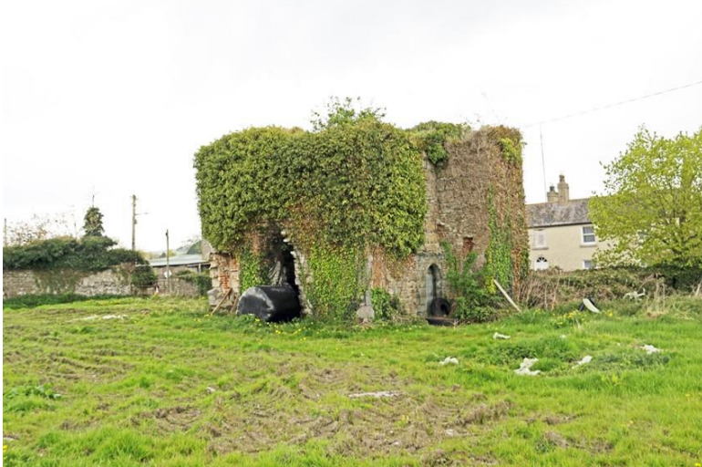
Figure 14.7 – Tower house to south of site entrance
