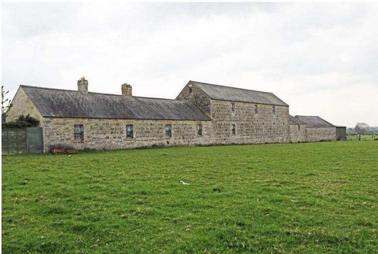
Figure 14.6 – Outbuildings at Newcastle Farm
